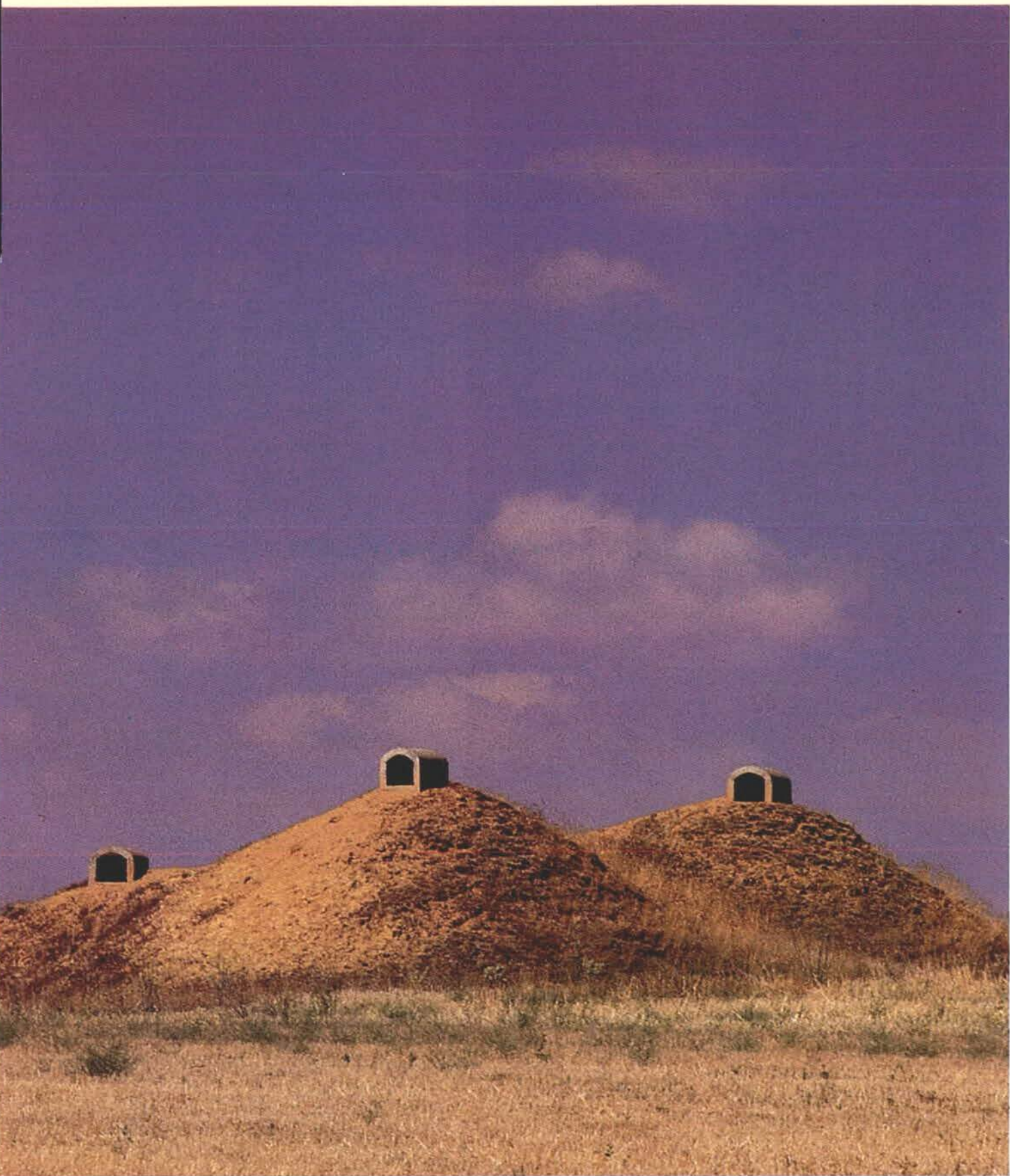
UNDERGROUND-BODEGAS. They are an ingenious way of preventing rain-water from seeping into the bodegas , allowing it instead to rundown the steep sides of the earthen mounds.
