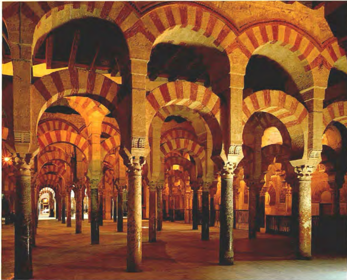
The mosque of Cordoba is unique and famous for its double arches supported on a veritable forest of columns.
