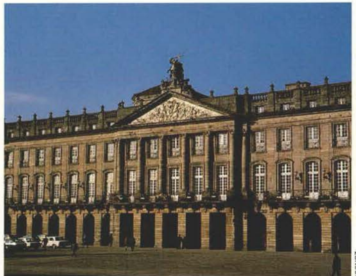
The splendid Palacio Rajoy in Santiago de Compostela is a good example of the neo-classical style.
