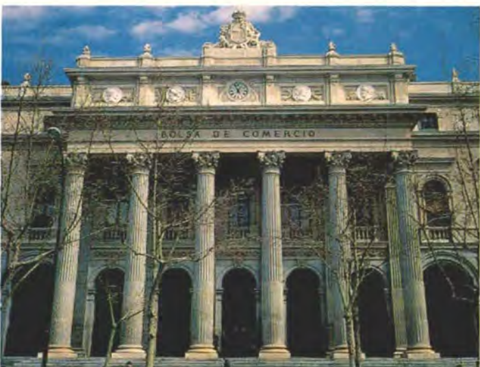
Madrid was one of the cities most favoured by the neoclassic style. Here, the Stock Exchange building.
