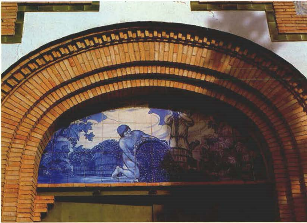
Masia Grabauc entrance portico features a brick semicircular arch which frames a decorative tympanum
