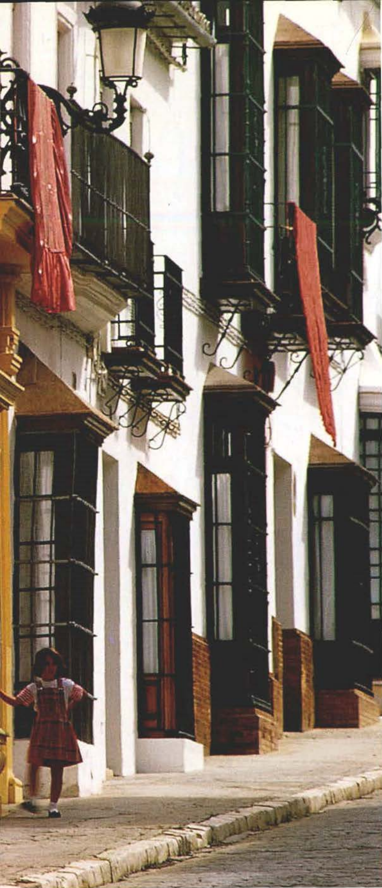
The windows in Osuna are all covered with grilles, standing out against the façade.
