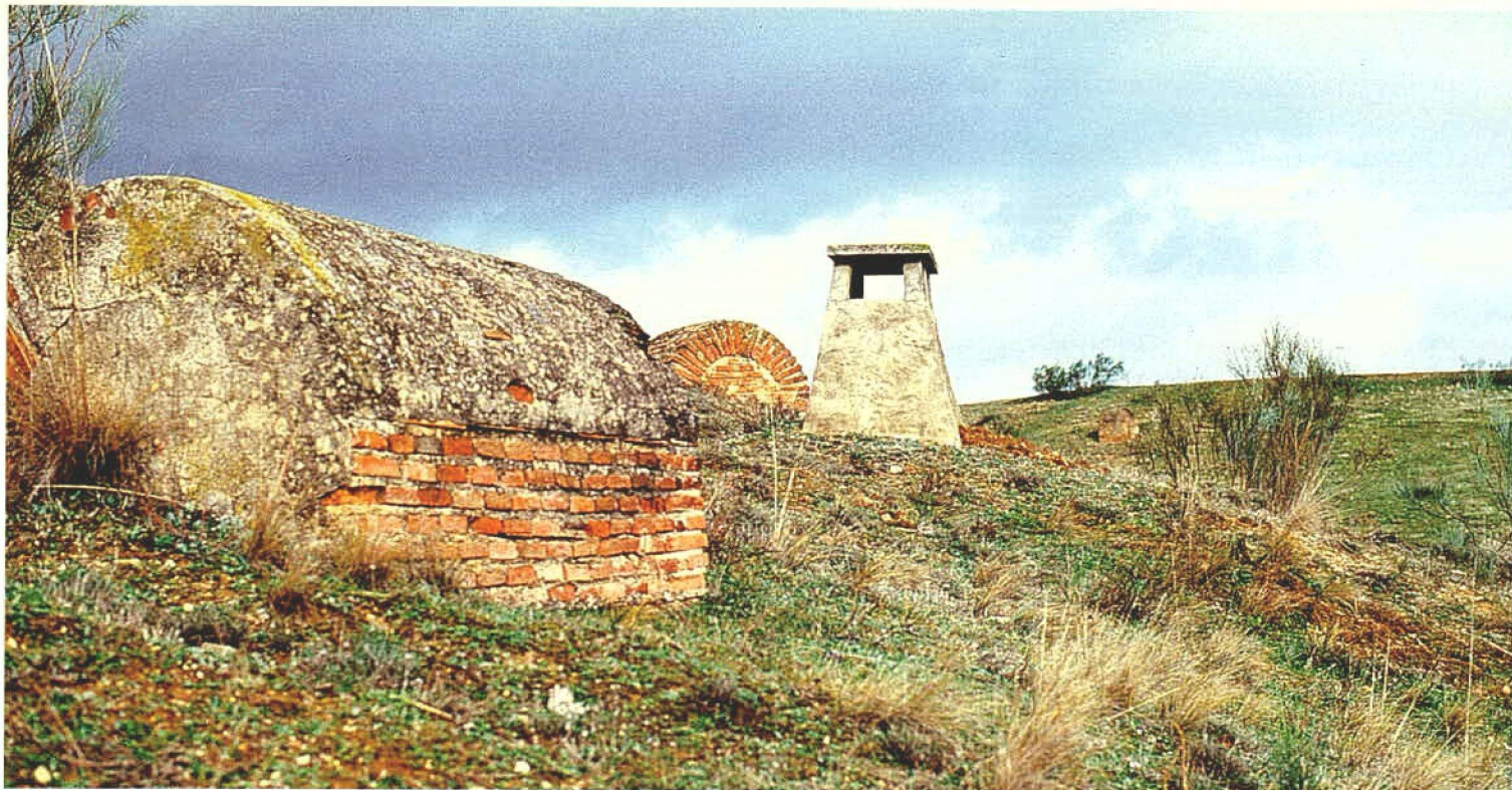
Subterranean aging cellars of Bodegas Antaño. Above: The typical luceras or zarceras ventilate this subterranean labyrinth
