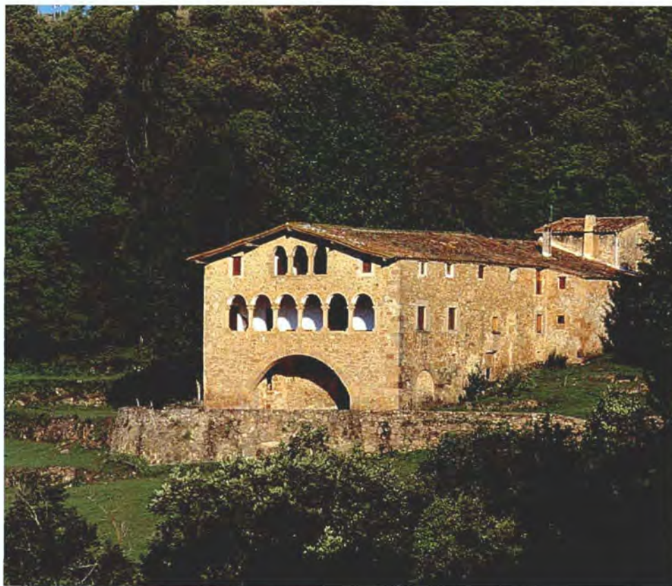
La Garrotxa's masias—the farmhouses characteristic of the Catalan countryside—are often imposing buildings, in both size and beauty.
