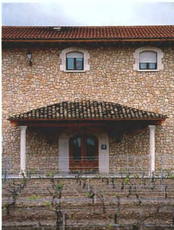
Top: Detail of the wine tasting room at Bodegas Torremilanos Bottom: Bodegas Arzuaga; main entrance to the hotel
